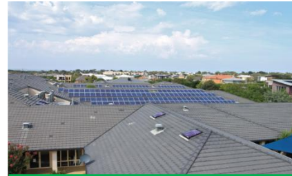
90kW Victoria, Australia
