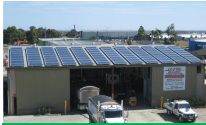
24kW Victoria, Australia
