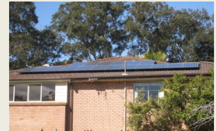
10 kW Newcastle, Australia
