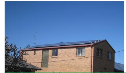
10kW Newcastle, Australia
